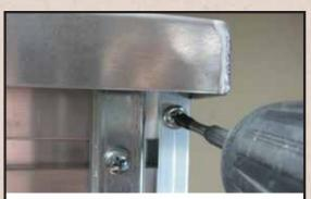
13. Install a DRILL POINT SCREW into each side molding on the back side near the top.
