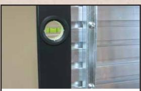
9. Install the other five SLATWALL PANELS using the same oreintation as the first (Fig. 7). Tap edge of panels with plastic hammer to align vertically. Tighten LONG PHILLIPS SCREWS on UPRIGHTS.
